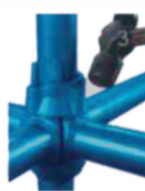
(3) Tightening with a hammer
